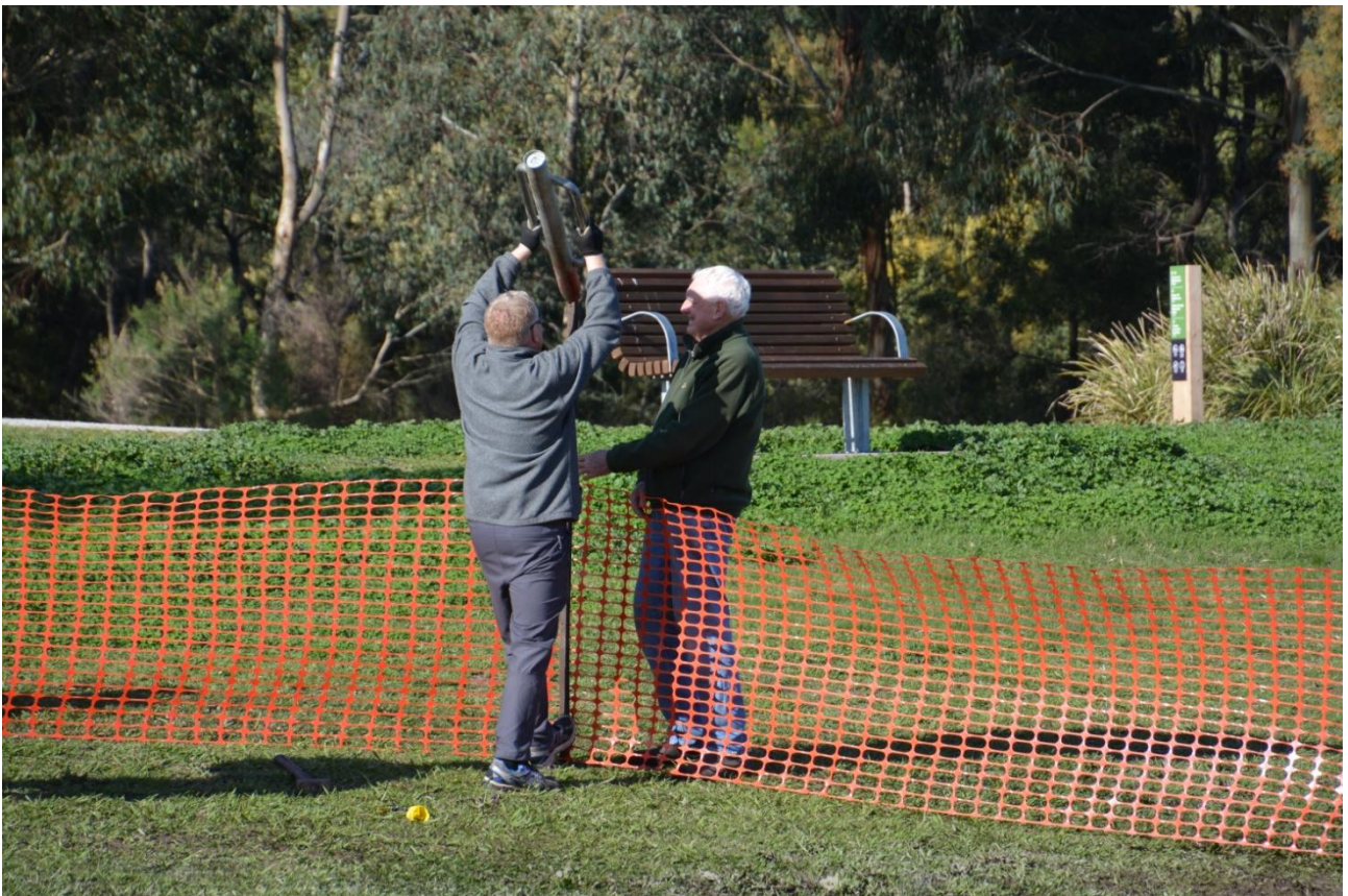
George and Lynton Erecting the Fence
